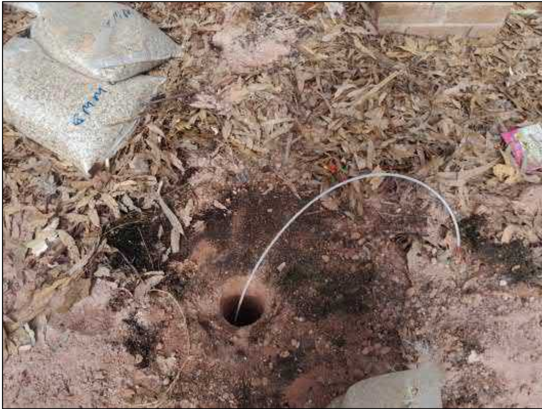
Photograph 7: Soil vapour well installation
