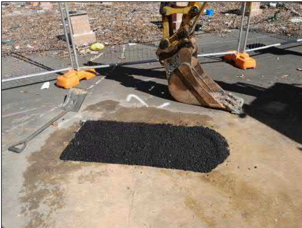
Photograph 16: Re-instatement including compaction and asphaltting undertaken at the completion of the investigation.
