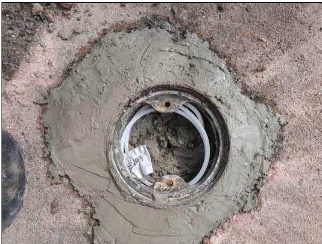
Photograph 9: Soil vapour well installation
