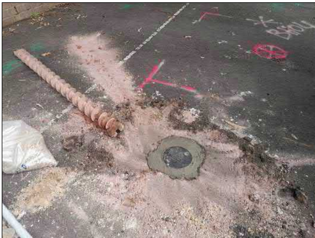
Photograph 10: Soil vapour bore installation completed with flush covers concreted into the ground and secured with bolts to prevent tampering and to allow sampling at a later date.
