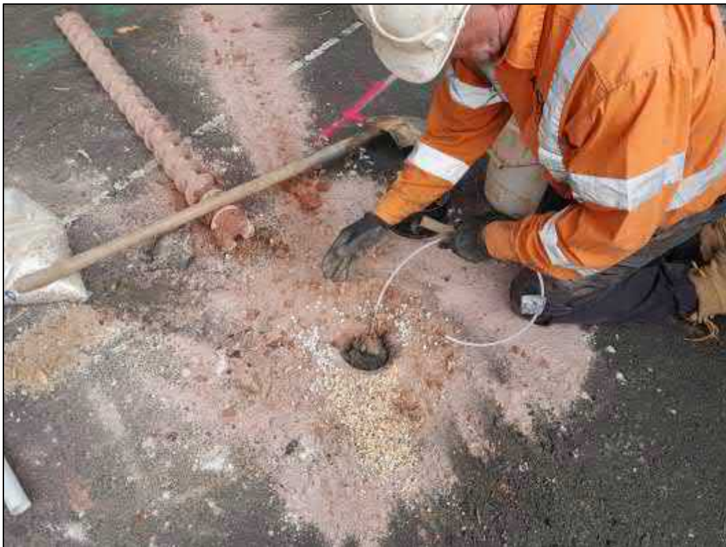
Photograph 8: Soil vapour well installation
